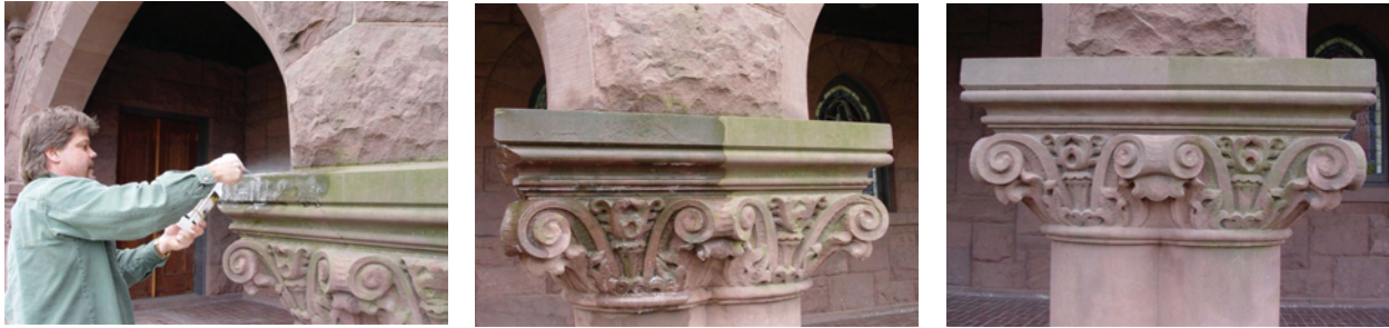
Biological growth removed with a single application of environmentally safe D/2.
